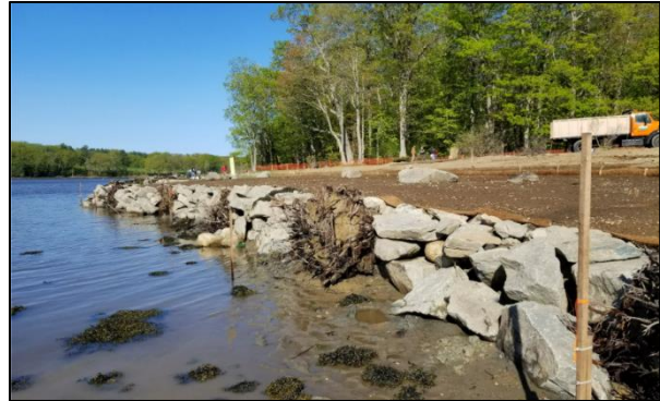
Rock sill and roots wads at Wagon Hill Farm Living Shoreline
