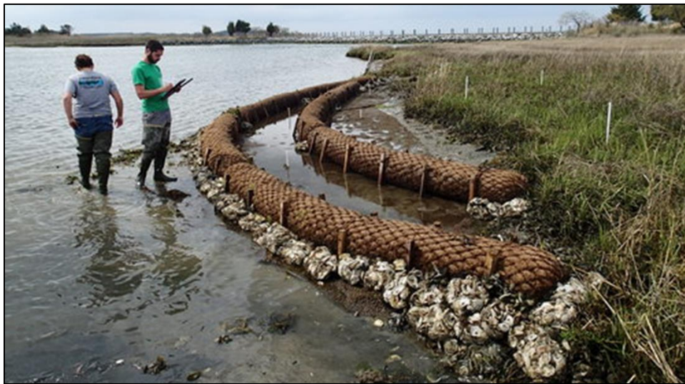
Example of an oyster shell and coir log shoreline treatment
