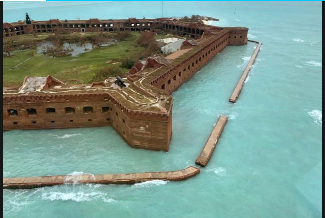
Fort Jefferson in the Dry Tortugas sustained storm damage as Hurricane Ian passed over the Civil War-era landmark on Tuesday, Sept. 27. A second section of the moat wall, at bottom, is among the new damage. The moat wall section at right was broken five years ago during Hurricane Irma.
