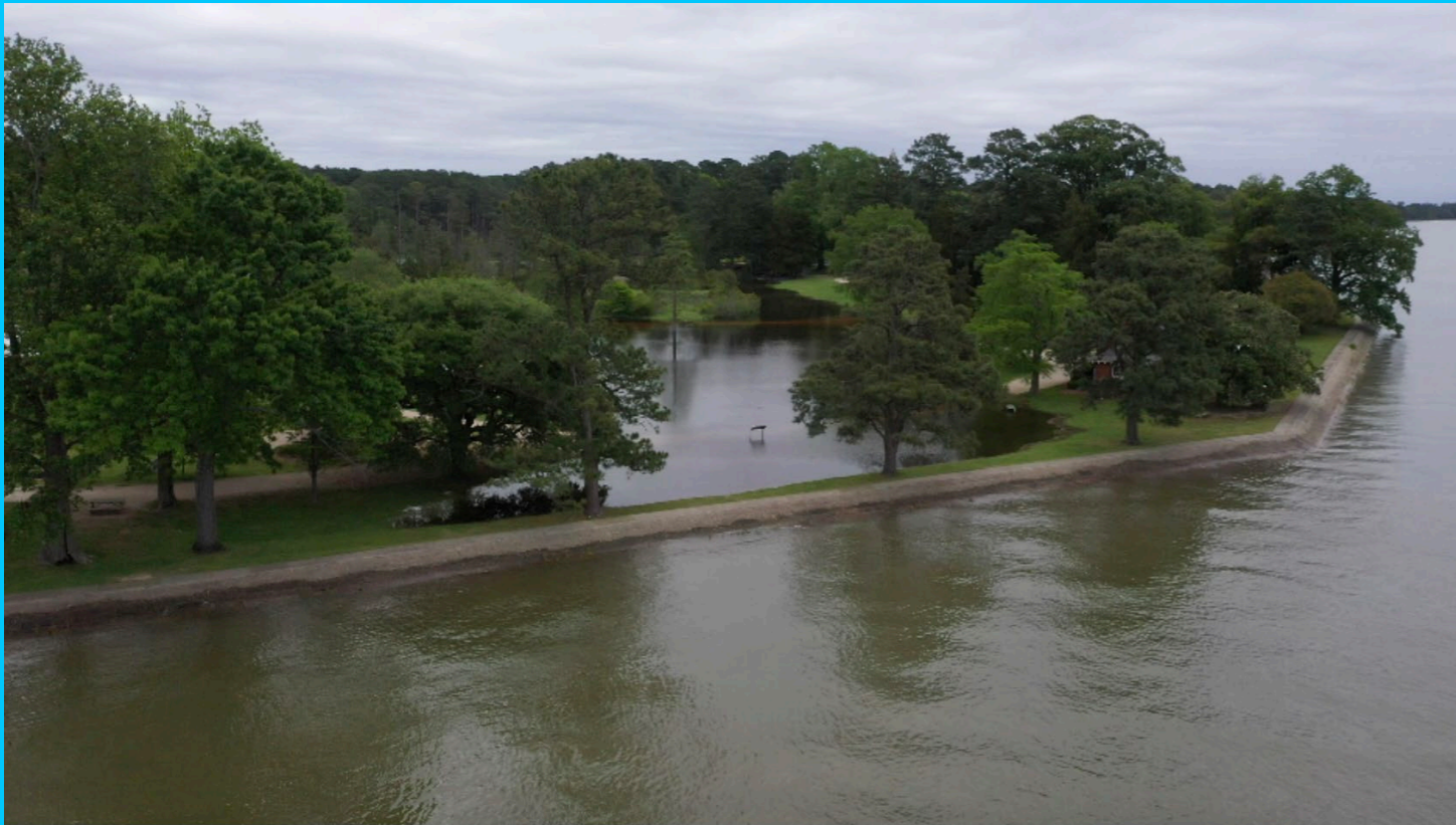
Despite its protective sea wall, Jamestown still experiences flooding. (Photograph courtesy of Jamestown Rediscovery Foundation/Preservation Virginia)
