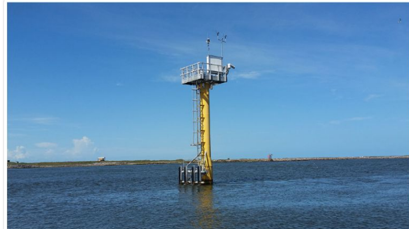
This NWLON station is specially reinforced to withstand hurricanes and other major storm events. The reinforced stations are better able to keep functioning during these events, providing critical information on water levels and winds that aids emergency response organizations.
